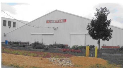
Helped Install Rain Garden & Rain Barrel at Marion Co. Fairgrounds w-RC&D grant
